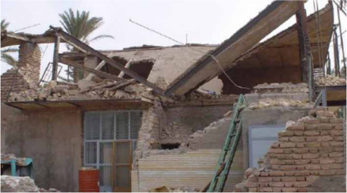
Bam earthquake in December 2003
