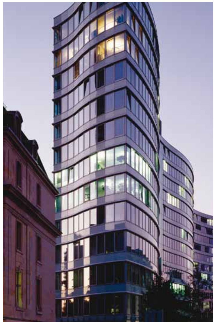
DIFA CitiQuartier Frankfurter Welle optimises energy consumption and cuts running costs with the help of Honeywell Energy Management Services
