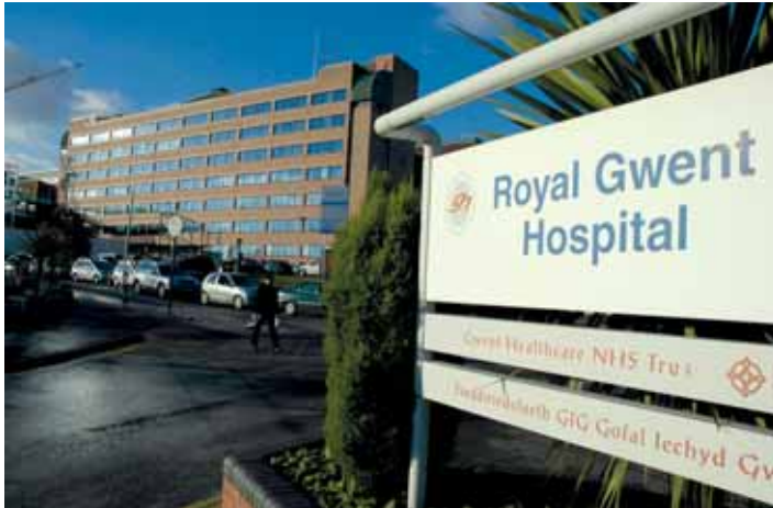
Figure 1. Royal Gwent Hospital saw savings of £1.5 million a year
